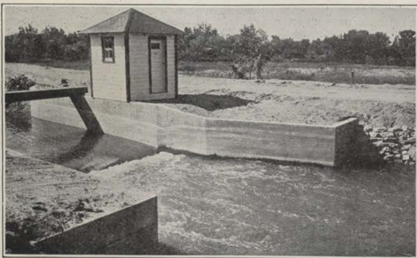
Twenty-foot Parshall Measuring Flume, for Bijou Canal, South Platte River Valley, near Greeley, Colorado.
