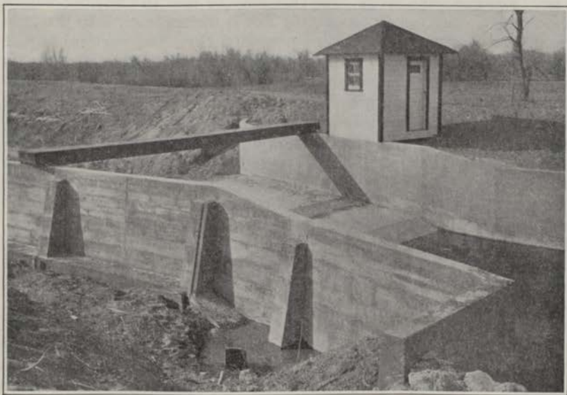
Figure 18.—Flume wall, with counterfort bracing, of the 20-foot flume on Bijou Canal.
