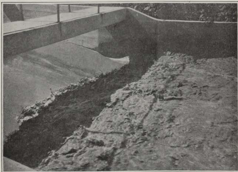
Figure 16.—A discharge of 550 second-feet passing thru the throat section of the 20-foot flume on the Holbrook Canal with 80 percent submergence. (See Table X.)
