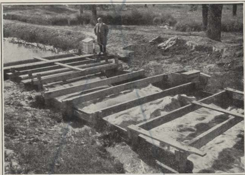
Figure 25.—Ten-foot Improved Venturi Flume Discharging 120 Second-feet Free-flow. Las Animas Consolidated Ditch, near Las Animas, Colorado.
