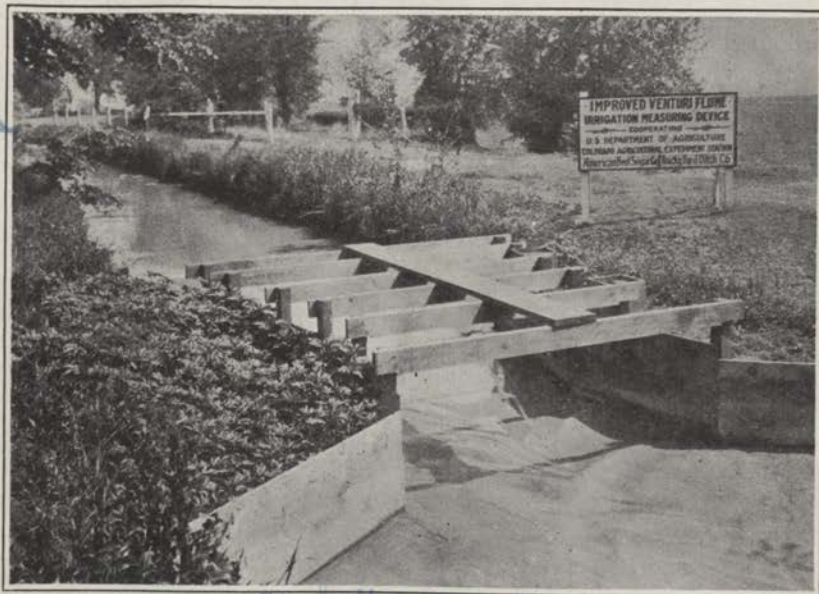
Baschall measuring Figure 9.—Six-foot Improved Venturi Flume Showing a Discharge of About 50 Second-feet with a Submergence of 95 Percent, Rocky Ford, Colorado.
