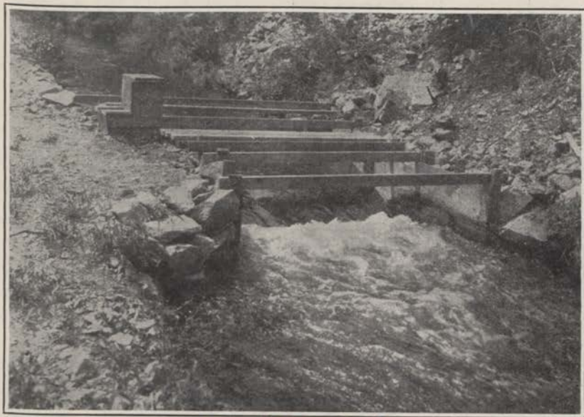
Figure 12.—Six-foot improved Venturi Flume Discharging 64 Second-feet with a Submergence of 60 Percent. Farmers' Ditch, Boulder, Colorado.
