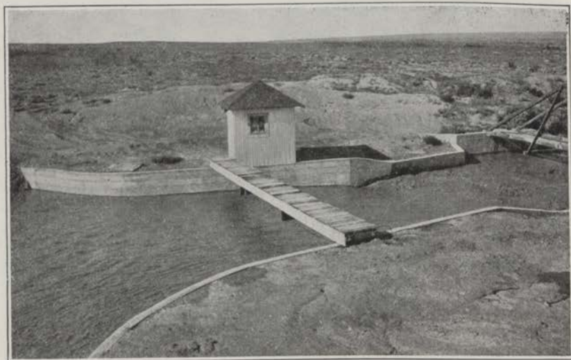
Figure 8.—Thirty-foot Parshall Measuring Flume, discharge 803 second-feet, submergence 89 percent, in Colorado Canal. (See Table X.)
