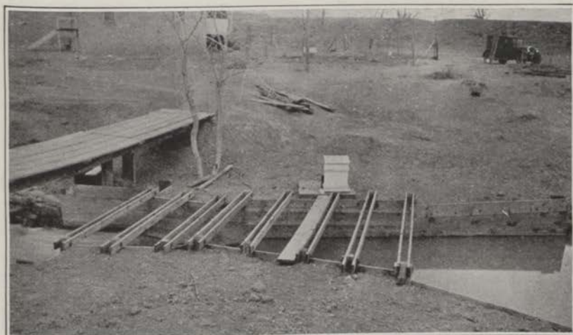
Figure 24.—Ten-foot Parshall Measuring Flume, discharge 27 second-feet, Fort Bent Canal. (See Table X.) In 1930 this was changed to a 14-foot flume.
